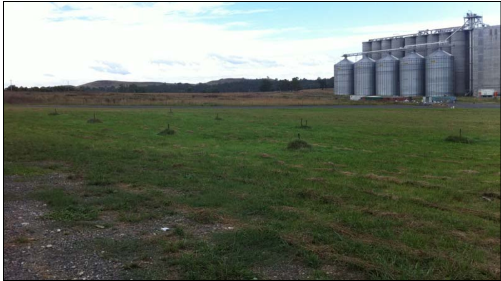
Figure 2: Allied Mills on-site effluent irrigation area (01.03.2011). 8 irrigation spray heads at 12m spacings. Mill in background.
